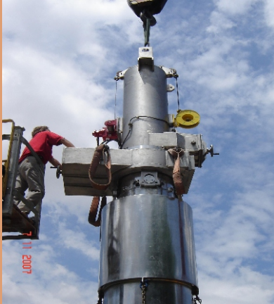
Figure 15. transportation of spent fuel elements
